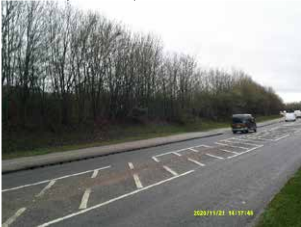
Shilo Way access point
